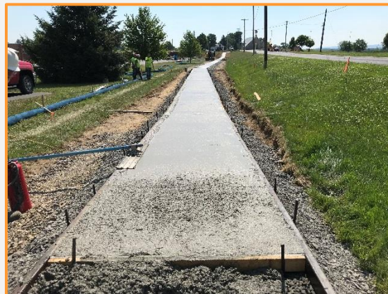
Ongoing sidewalk construction along Mount Rock Road to connect the High School to the Middle School
